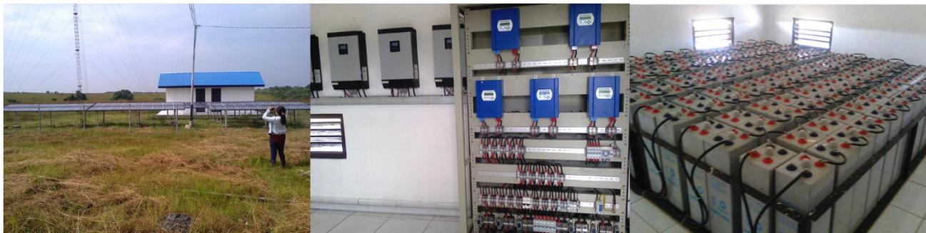
Figure 5.3. (Left) 13.5 KWp PV power plants for local transmigration location (Center) the systems (Right) batteries.
