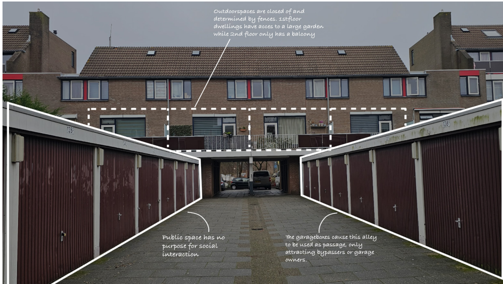
Observational analysis shows that this neighbourhood has no social facilities or functions. Interaction between residents could only occur near their own dwellings.
