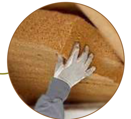
Adding insulation wood wool
