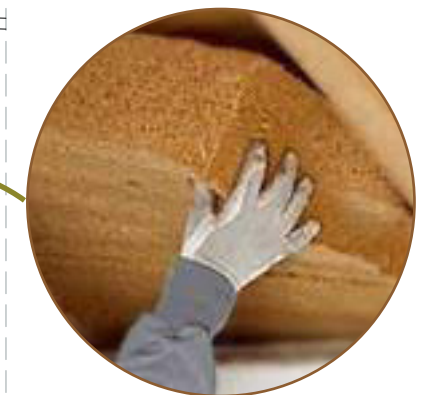
Adding insulation wood wool
