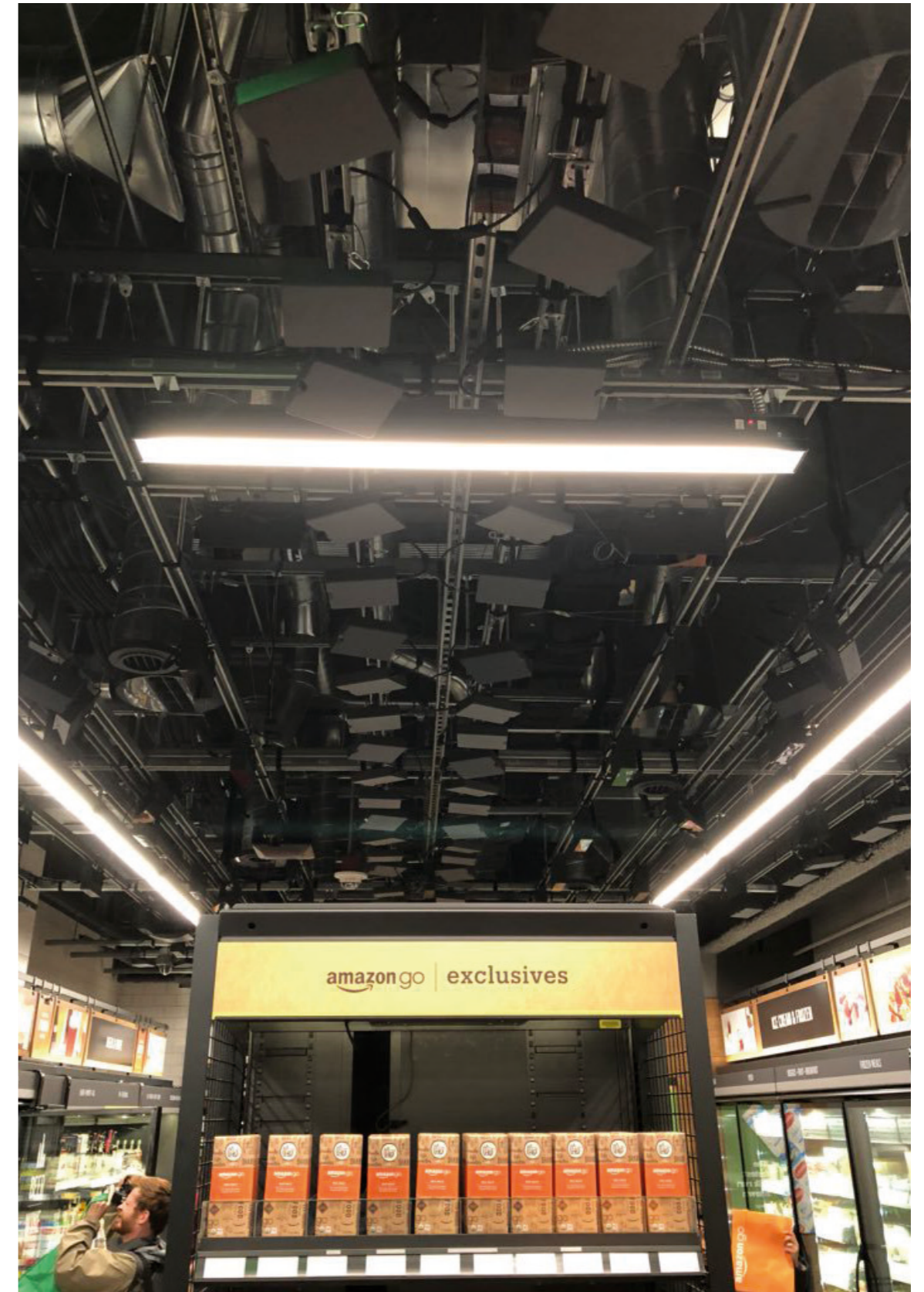
The ceiling of Amazon Go is splattered with cameras [Photo : Tom Rubin]
