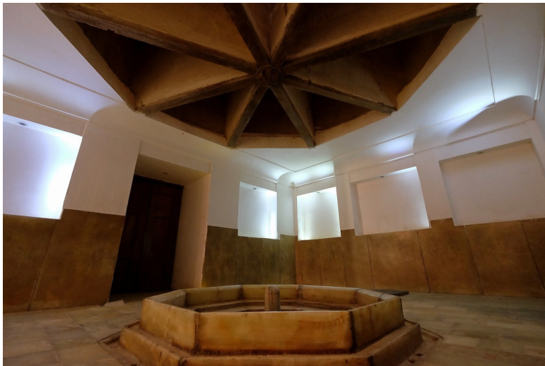
Figure 5.3. The opening of a wind tower ending above a fountain to increase the evaporative cooling.
