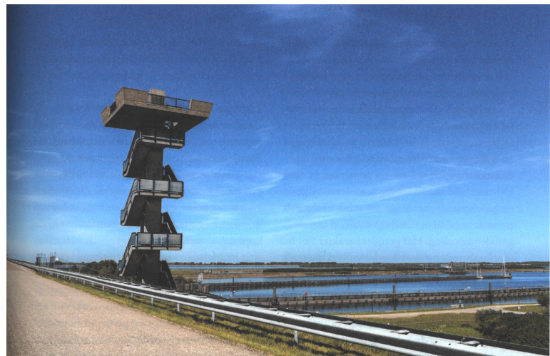
Figure 6.11. The watchtower on the Philipsdam, providing a wide view of the surroundings.
