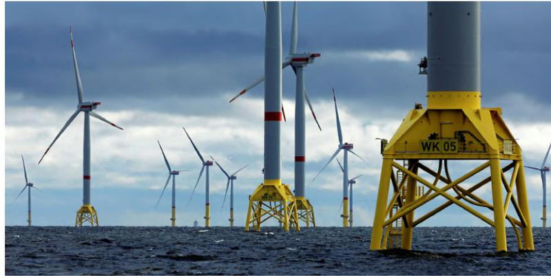
**Figure 1-4:** Wikinger jacket, x-braces omitted at sea level
