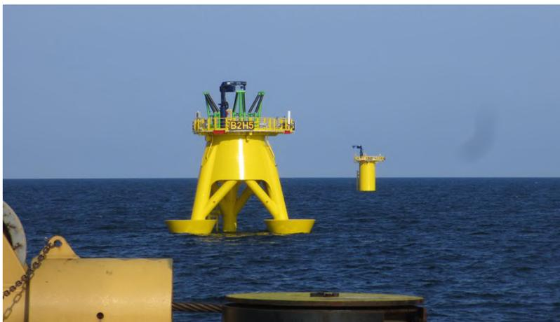
**Figure 1-3:** Baltic 2 jacket, ice cones installed at legs
