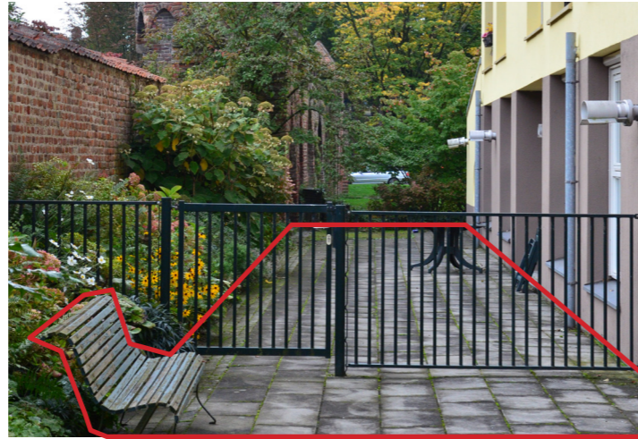
poor relation between city wall and building
