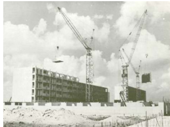
Figure 2. Cranes to build higher modular buildings (BouwhelpGroep advies en architectuur, 2013, p. 19).
