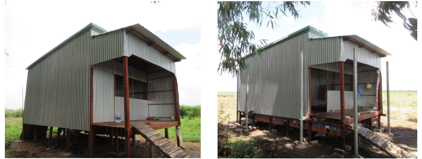
Figure 77. Stilt homes in Vietnam Mekong Delta converted to Amphibious homes with local materials (Vietnam n.d.)
