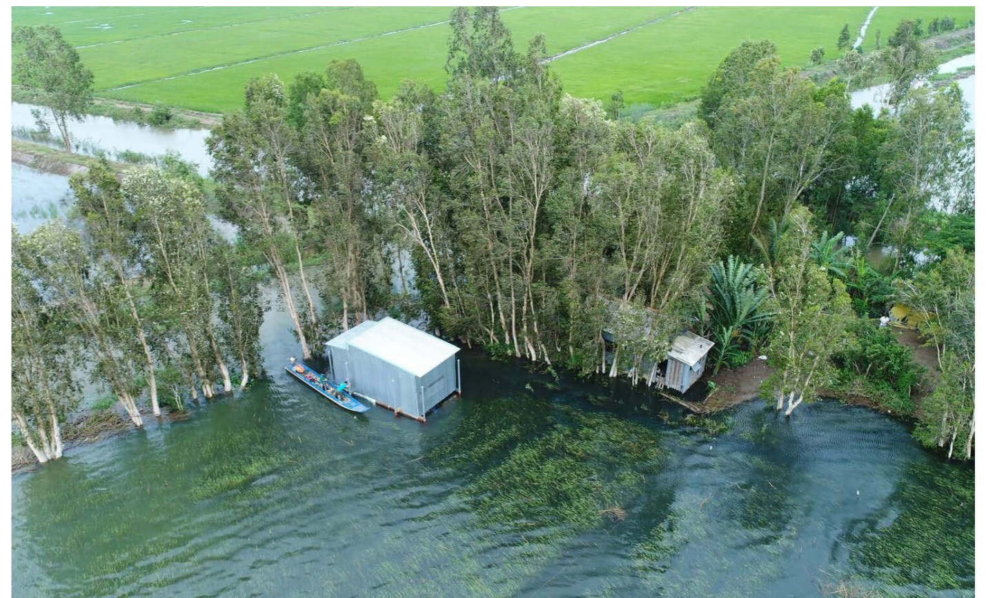
Figure 78. Retrofitted Amphibious homes during floods in the Mekong Delta (Vietnam n.d.)
