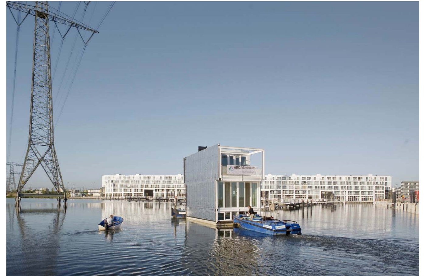
Figure 55. Prefabricated units being transported through the canals and placed on site (Waterwoningen ,2015)
