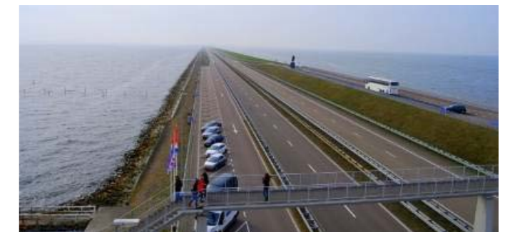
Figure 46. Closing of Zuiderzee project in 1932 with a dam Afsluitdijk at IJsselmeer (Nillesen & Singelenberg, 2011).
