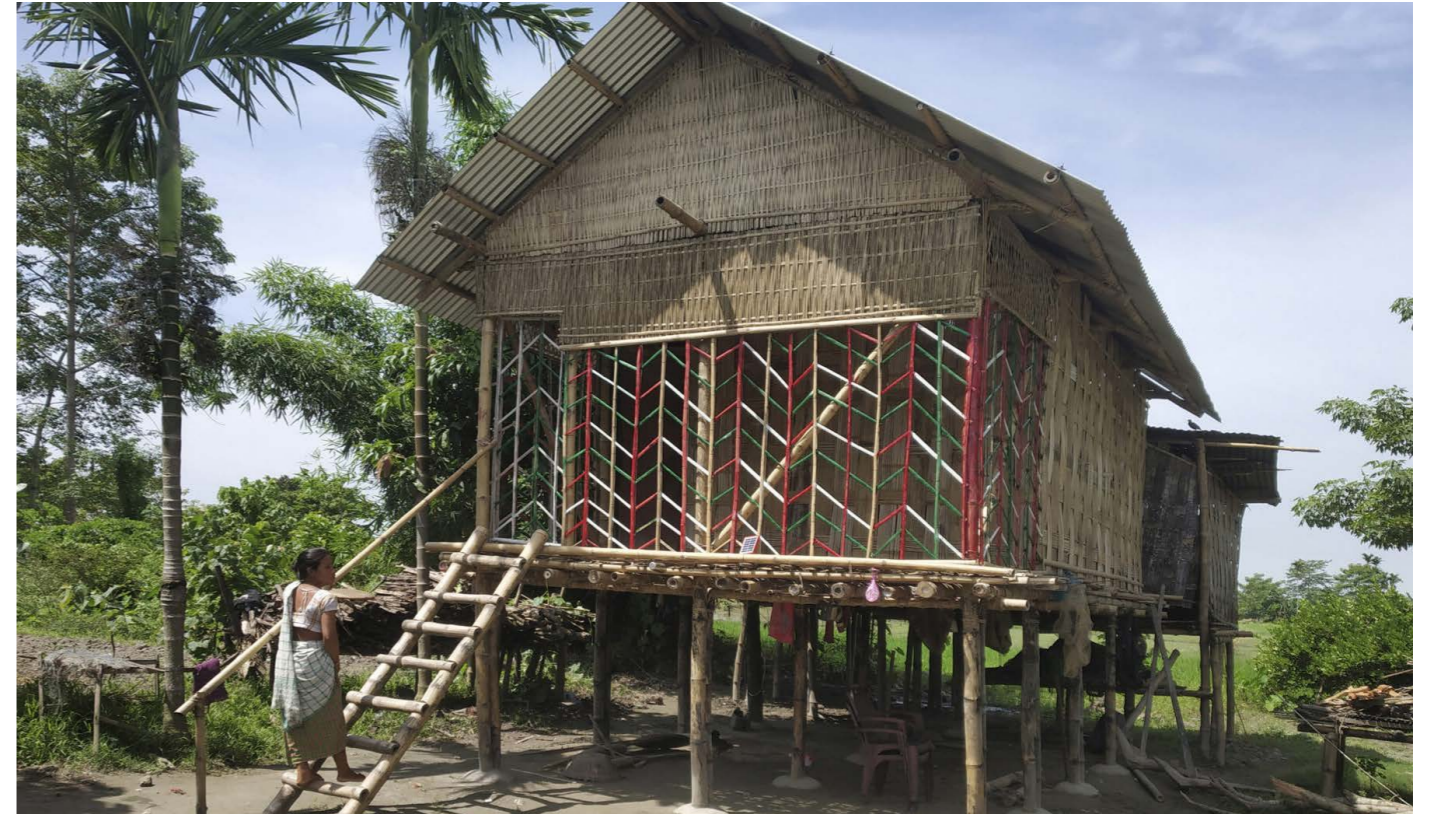
Figure 75. Chang Ghar from Assam India, standing on wooden stilts being accessed by a ladder. (Krishna, 2023)
