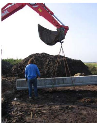
Figure 11 Foundation strip positioning
