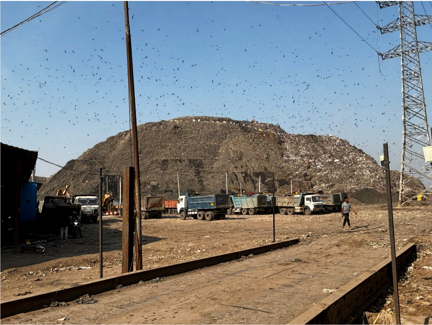
Fig 1. Ghazipur landfill, East Delhi
