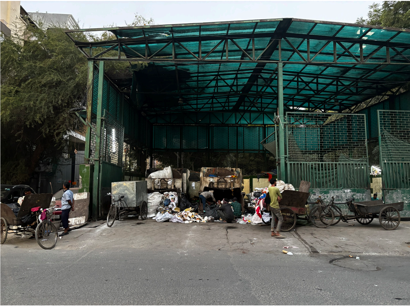
Fig 12. Fixed compactor transfer station, West Delhi
