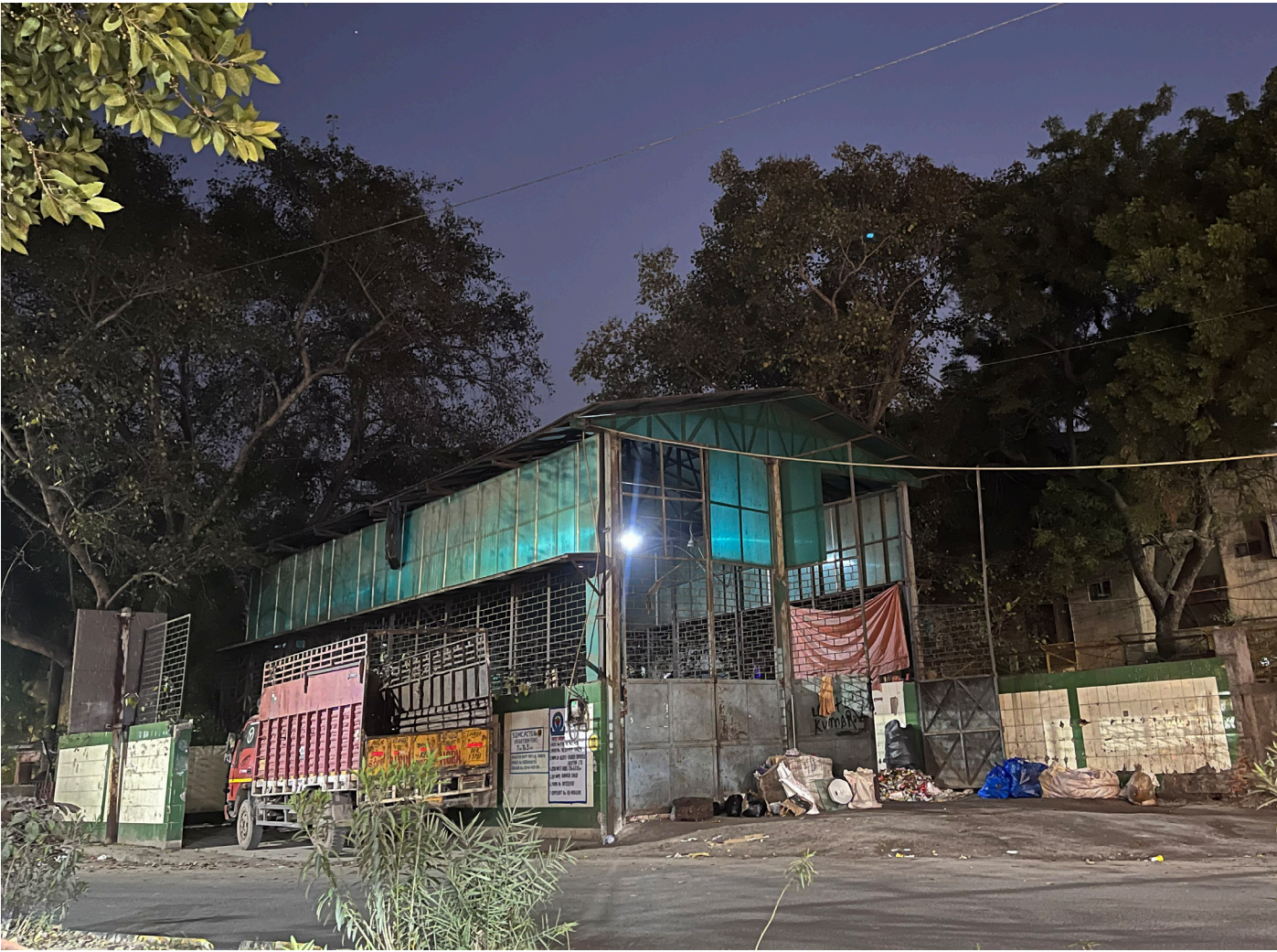
Fig 13. Fixed compactor transfer station, West Delhi
