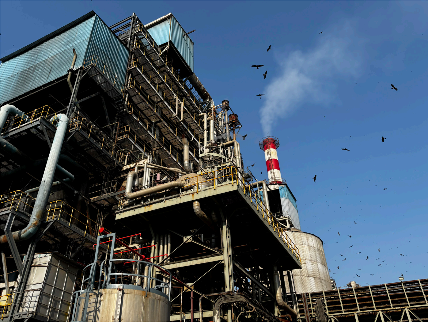
Fig 2. Incineration (Waste to Energy Plant) near Ghazipur Landfill, East Delhi
