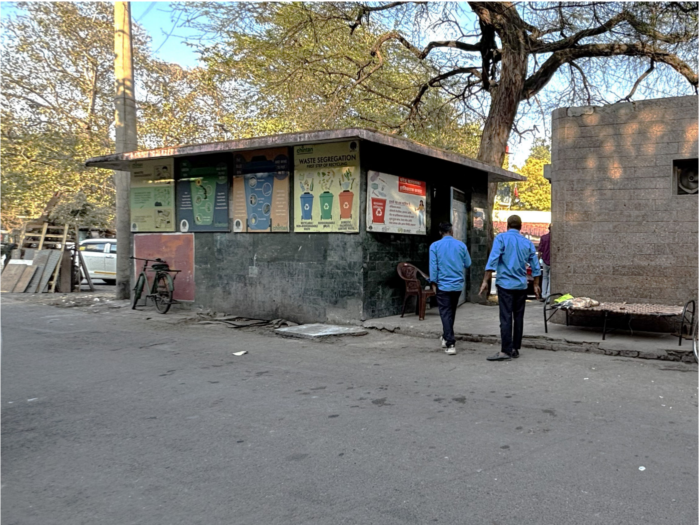
Fig 5. Material recovery facility on a neighbourhood street, New Delhi
