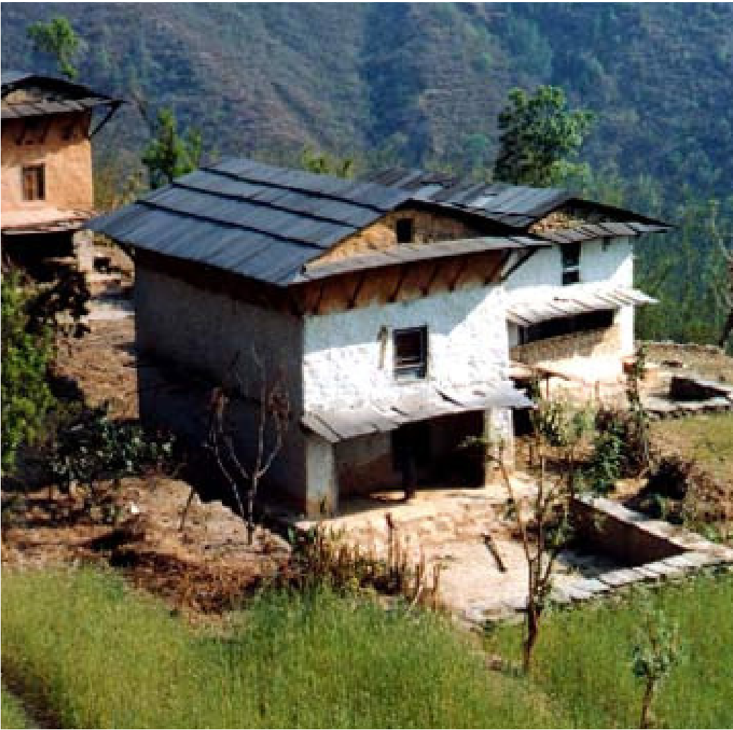
Sherpa House courtesy of Photo Voyages. Steep roof, roof overhang on two levels , small windows, retaining wall made out of stone in back garden, along with trees and plants to prevent soil erosion.
