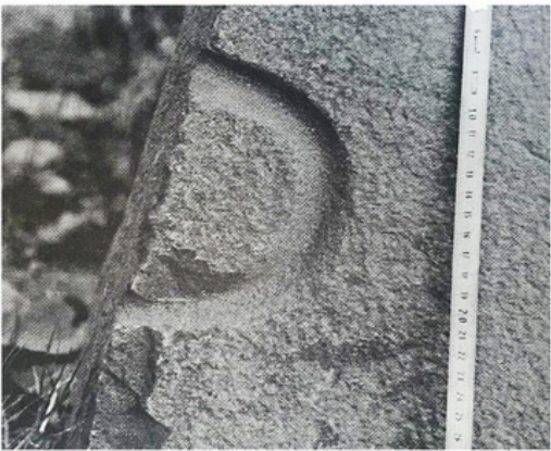
T-shape and U-shape notches in rocks found in Ollantaytambo. Image courtesy of Jean-Pierre Protzen.
