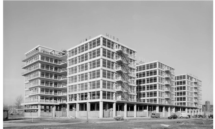
Figure 06A.3: External vertical circulation
