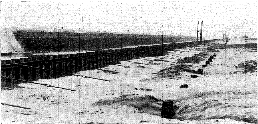
FIG. 37.—STEEL SHEET PILED RIVER WALL.
