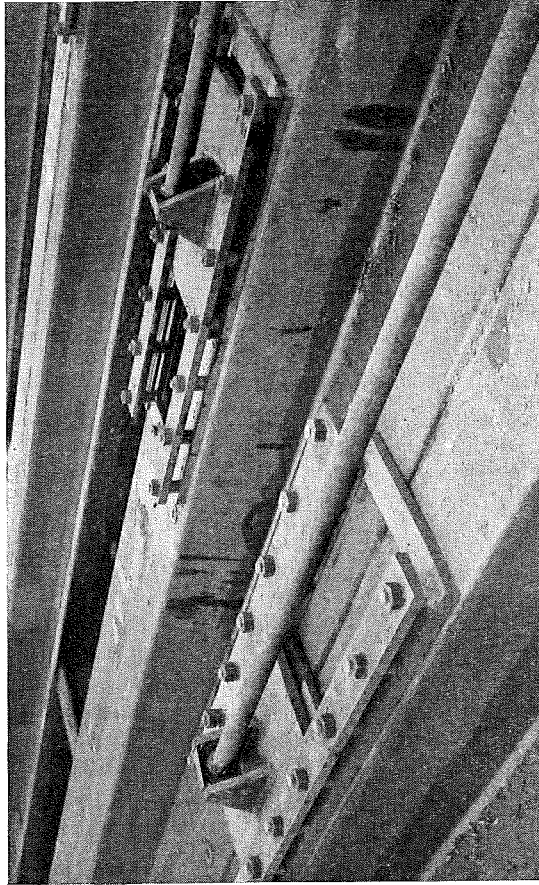
FIG. 64.—SLUICE GATES IN STEEL SHEET PILES.
