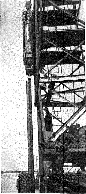
FIG. 17.—DOUBLE-ACTING STEAM HAMMER USED WITH PILE FRAME.
