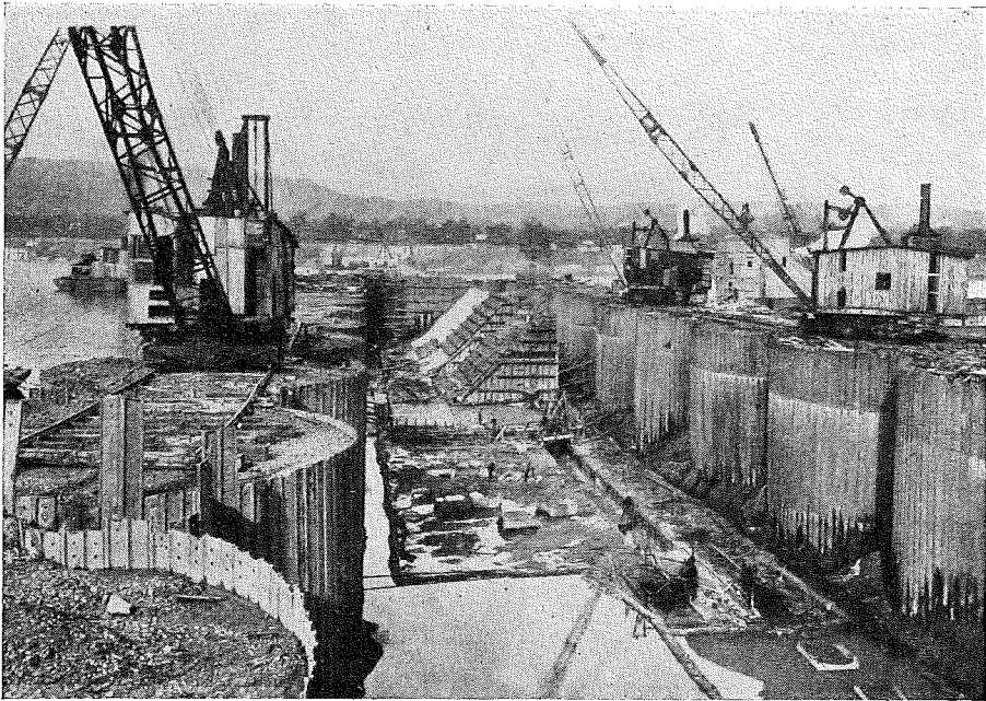
FIG. 82.—CELLULAR COFFERDAMS.
