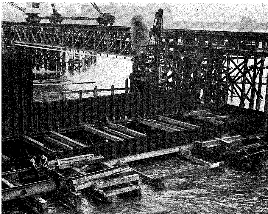
FIG. 87.—COFFERDAM FOR PIER OF WATERLOO BRIDGE, LONDON.
