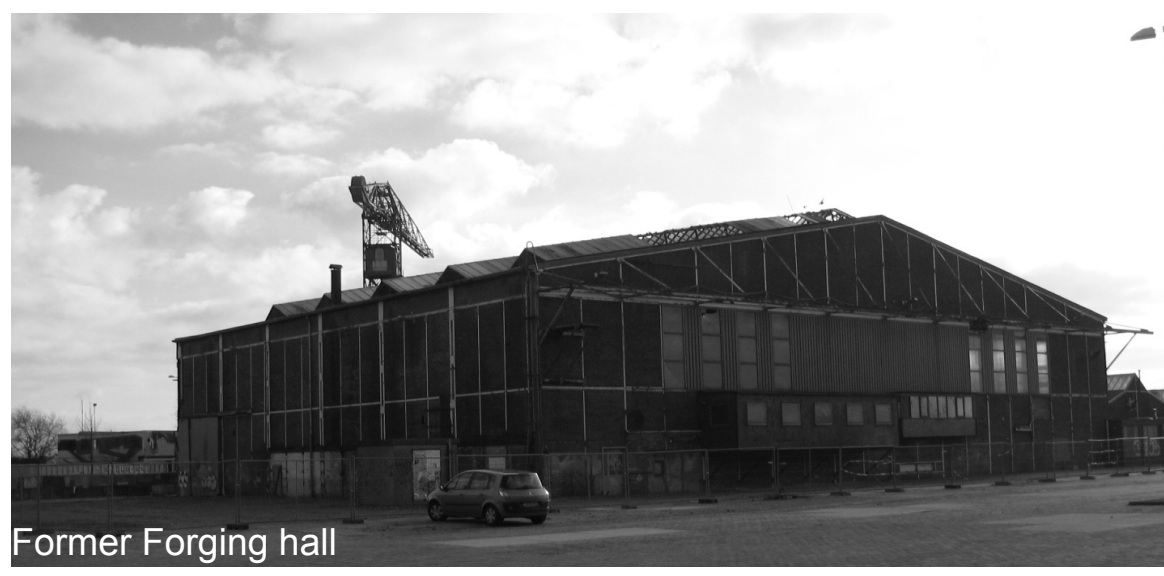
Former Forging hall
