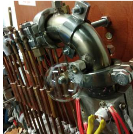
(b) The leak in the PEEK-Nail electrical pass-through after getting subjected to high temperature.
