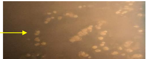
Figure 97b Full-scale RSF during ETSW bed, spouting channels
