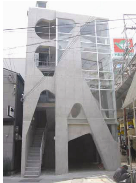
Fig. 5.14. Inside views and outside views of the completed building [27]
