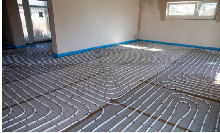
Figure 4.21: Picture of pipes laid on the floor to provide underfloor heating in the room, Verbeterjehuis.nl (2024)
