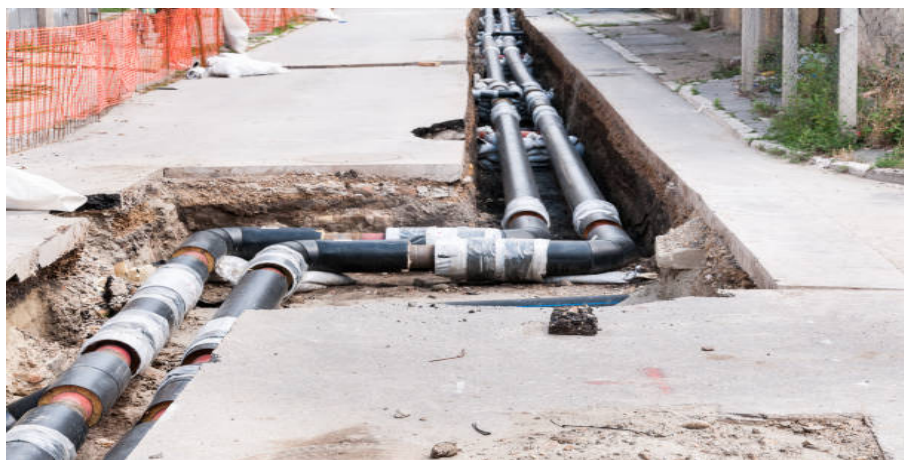
Figure 4.26: Laying of pipelines underground to connect aquifers and buildings, Getty images
