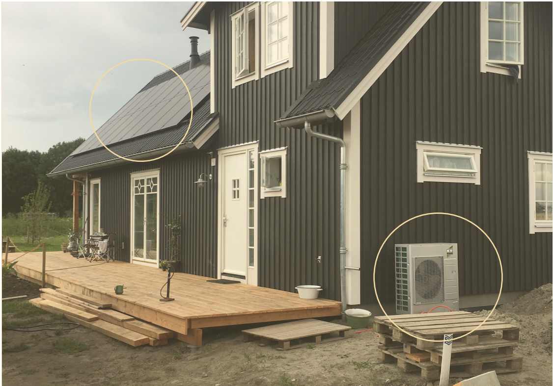
J. Photovoltaic panels and a heat pump (photo by author, Oosterwold)
