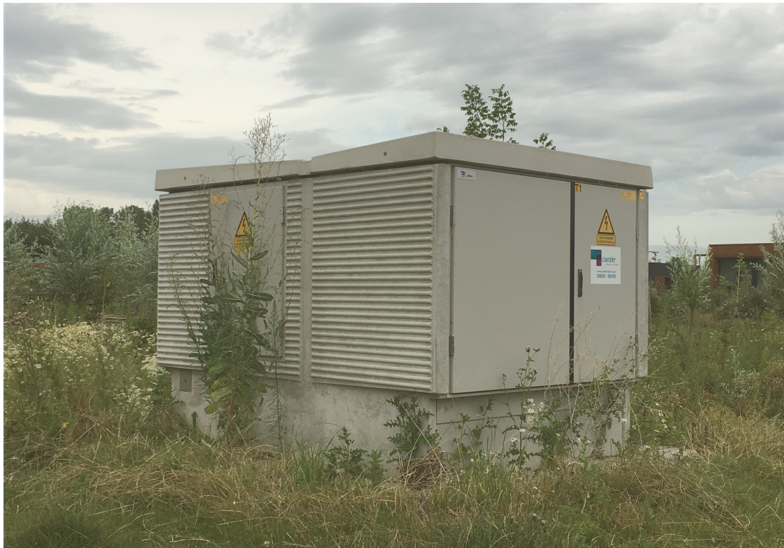
K. Transformer to connect households to the national electricity grid (photo by author, Oosterwold)
