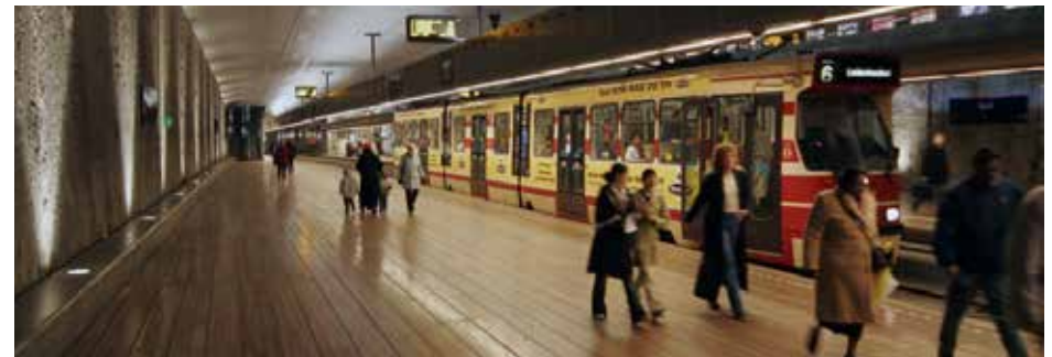
Figure 1-4: Tram tunnel, The Hague (IGG, 2014)
