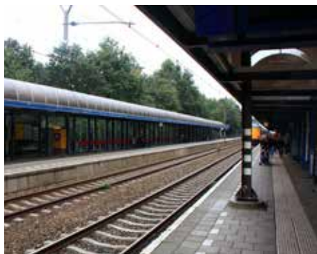
Figure 6-20: Rotterdam Alexander train platform
