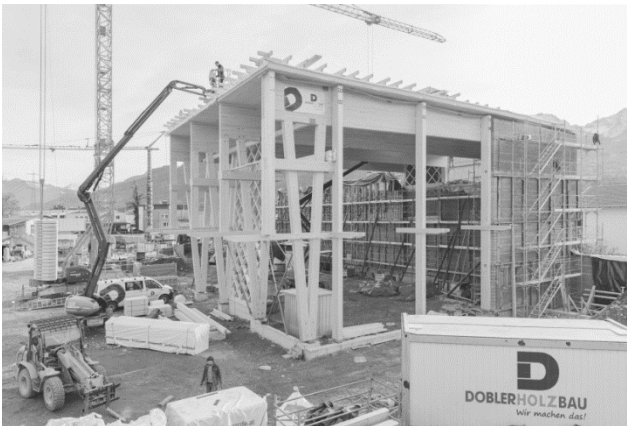
Fig.: 9, Source: (Rauch, 2019) ERDEN, production hall for prefab rammed earth components, Schlins, Austria
