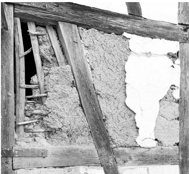
Fig.: 7, Source: (Laimer, 2020) Traditional sub construction for the straw clay infill of a half-timbered house.
