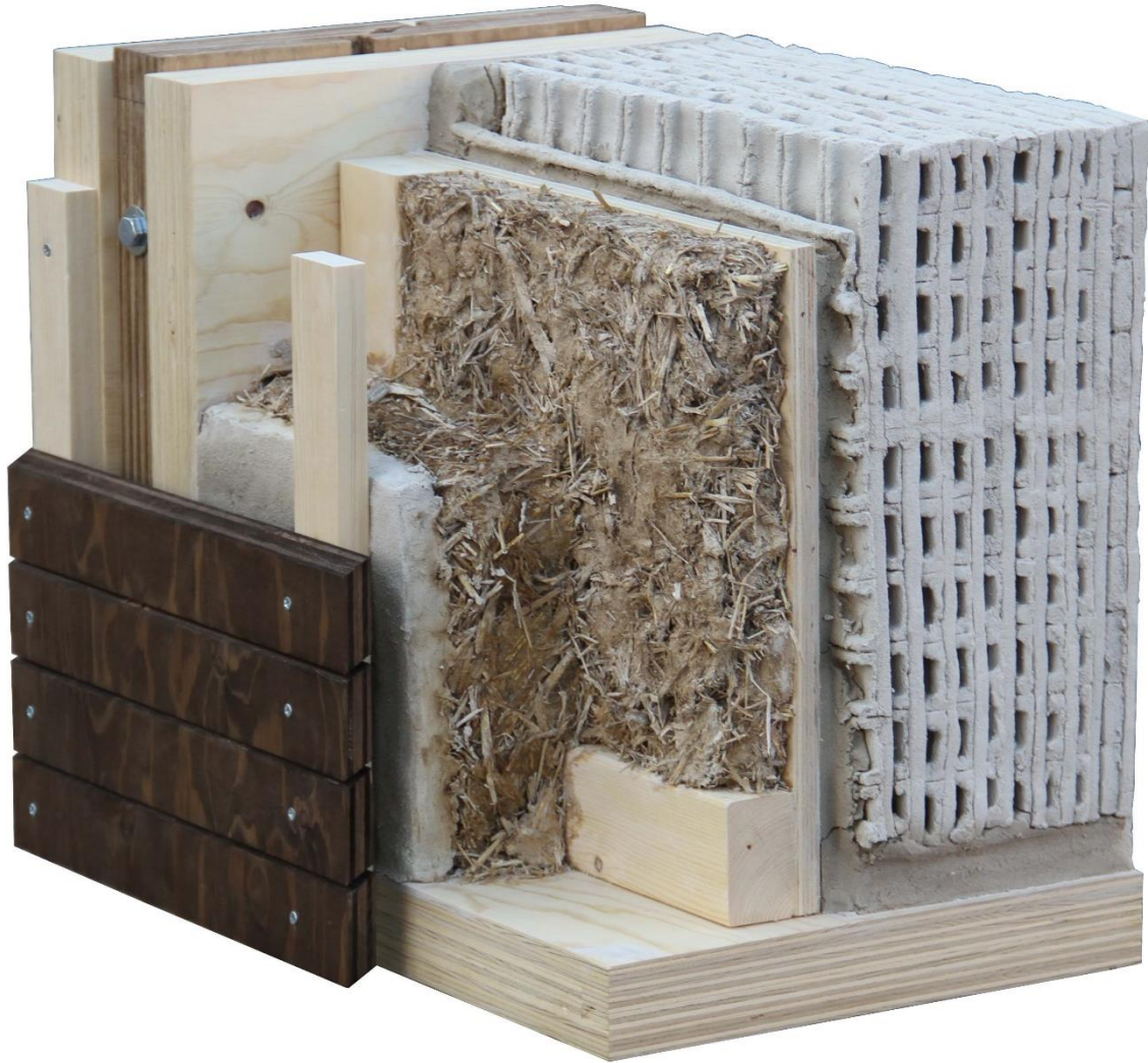
Fig.: 956, Front view, charred cladding, clay covered straw insulation, spacer, 3DPE gradient infill.
