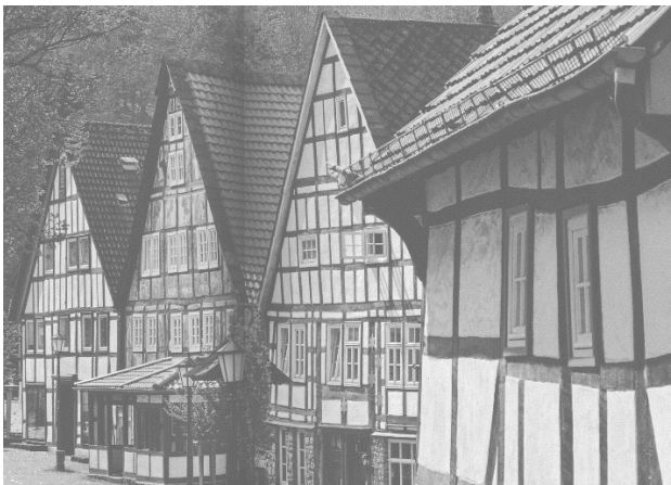
Fig.: 6, Source: (Dethier, 2019) traditional German half-timbered house. The timber skeleton carries the weight of the light earth infills. The infills are a mixture that contain high amounts of straw and other fibres to reduce the weight and increase the insulation.
