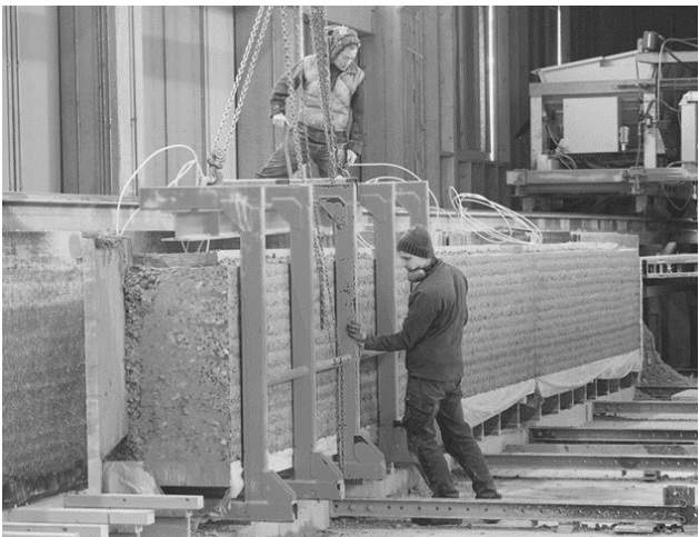
Fig.: 10,Source: (Rauch, 2019) Assembly of a prefab, monolithic rammed earth wall. Schlins, Austria
