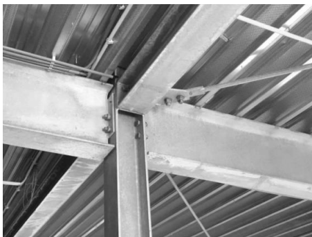
Figure 60. Structural elements and connections in The Green House (Doomen, 2018)
