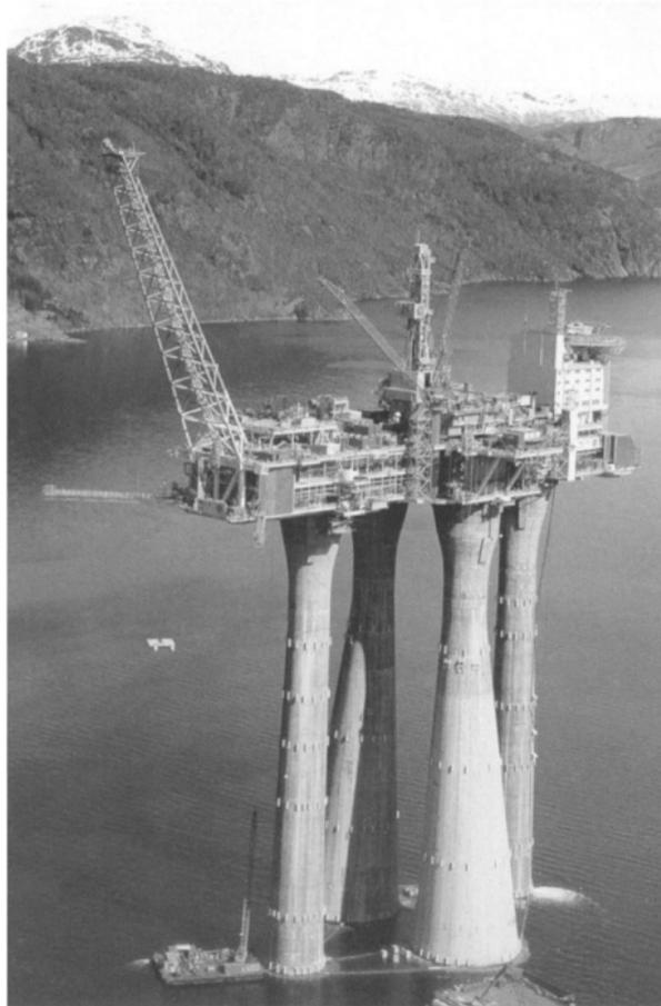
**Figure G.2:** Towing of Troll A platform to its final location [93]
