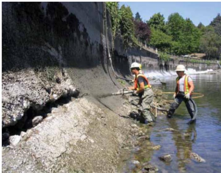
**Figure F.4:** Shotcrete application in the repair of a concrete face [75]
