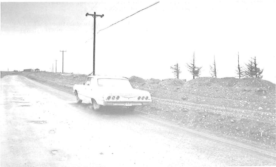
Photo No. 5 - This was taken in June 1965 and shows the new berm being built up 500 feet down drift from the groin area. The spruce trees in the picture have been killed by the salt water.
