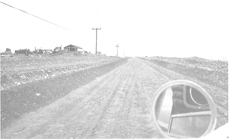
Photo No. 4 - June 1965. Shows the highway on Spit where combinations of high tides and waves have deposited material in a new berm. The Highway Department removes the material by either plowing to the side or banking it to another location.
