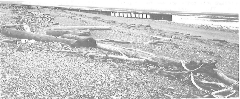
Photo No. 2 - June 1965. Shows the timber groins as opened up by cutting with a chain saw.
