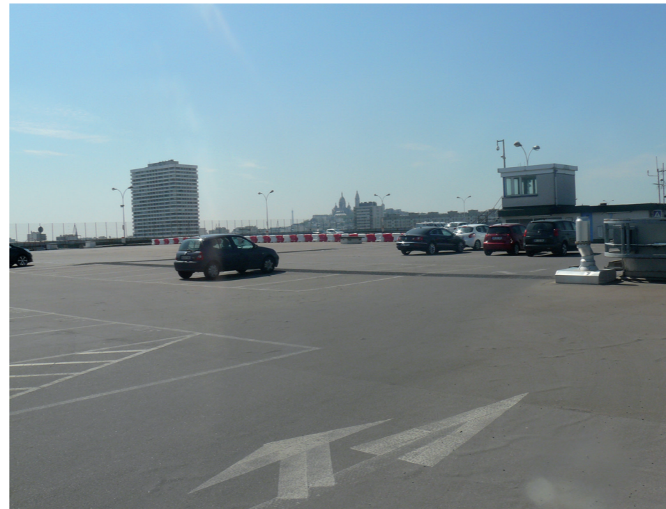
Parking deck, view on Sacre Coeur
