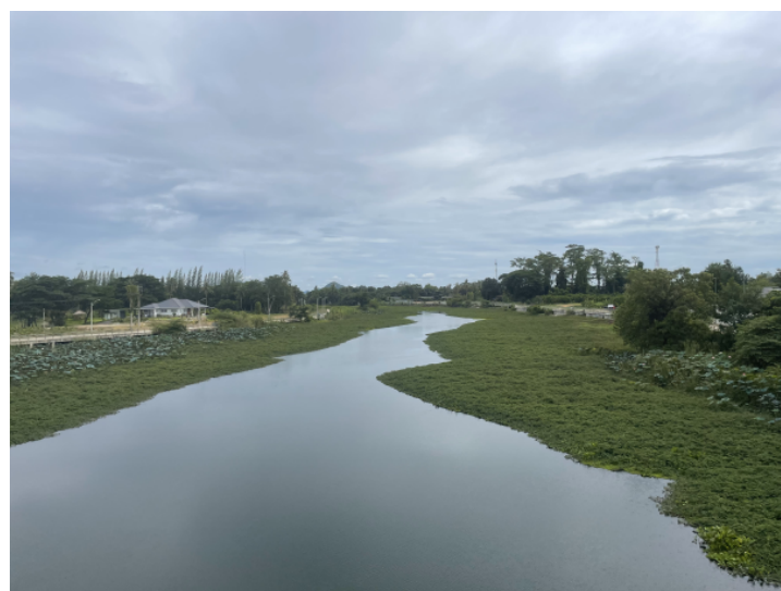
Figure 2.4: Phetchaburi river around 1 km upstream of the Phet Diversion Dam.
