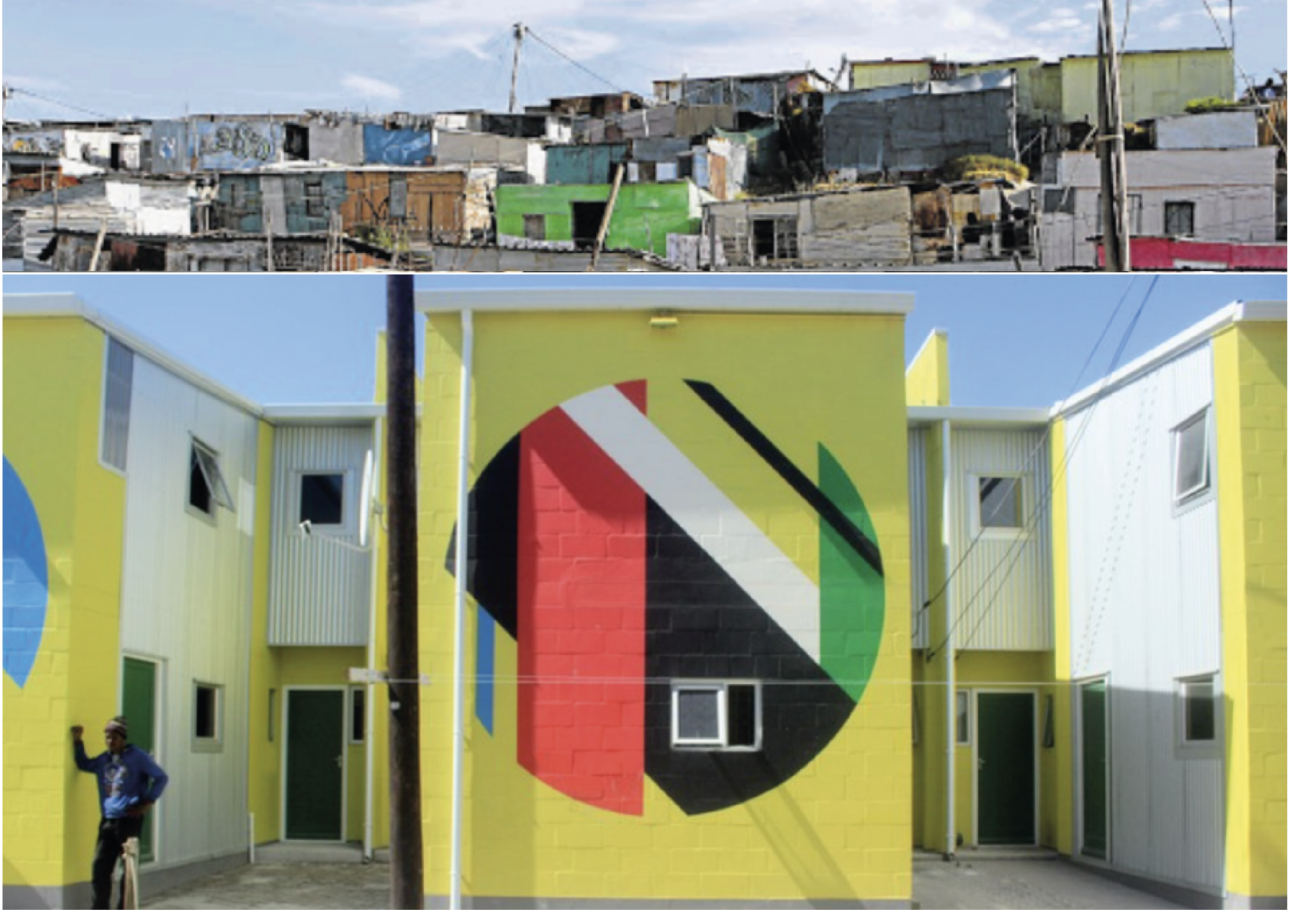
Figure 6.29: This is a picture of the Empower Shack project when it was first completed. It is built partially with brick and timber clad in corrugated iron. Reference: https://groundup.org.za/article/73-families-move-into-newly-built-alternative-affordable-housing-models-in-khayelitsha/
