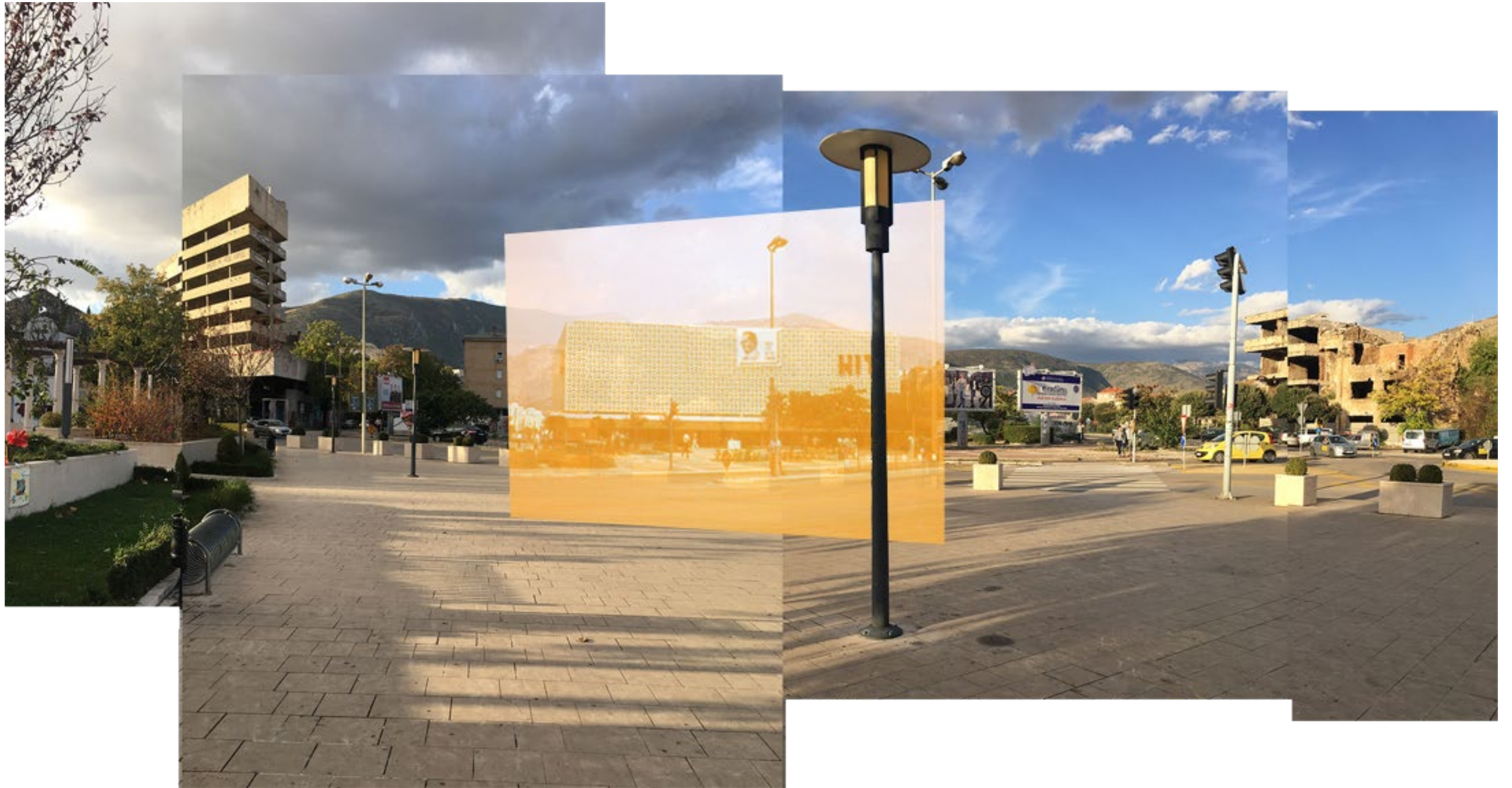
View of former HIT site from the 'Spanish Square' (location of HIT shown)
