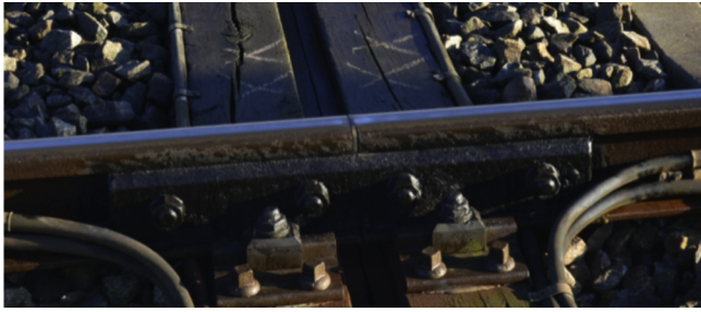
Fig. 21. Typical IRJ in the Dutch railway network.
