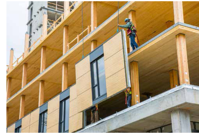
Composite Timber - Concrete Slabs CLT Beam & Columns
