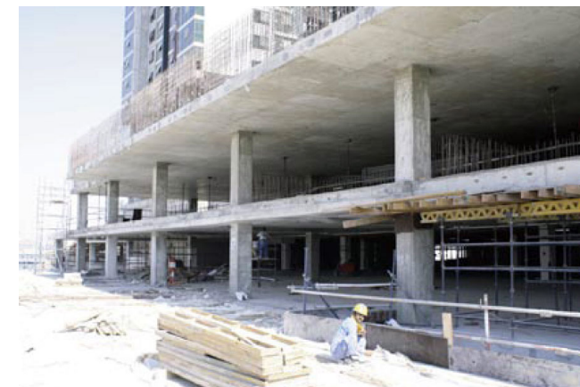
Concrete Flat Slab Construction
