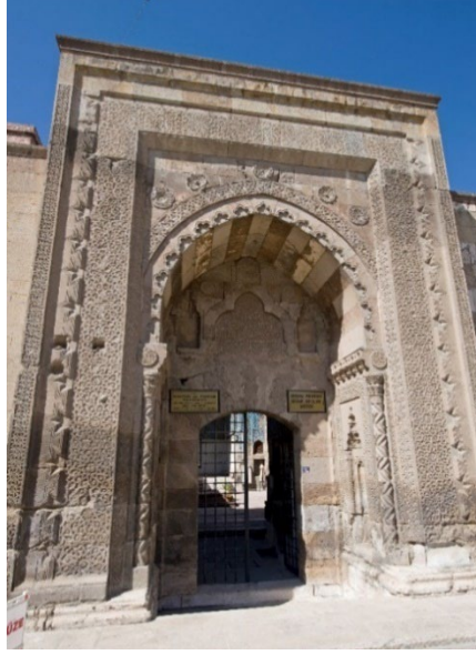
Figure 3 Sircali Madrasa – Façade (Okur Yazarim, 2017b)
