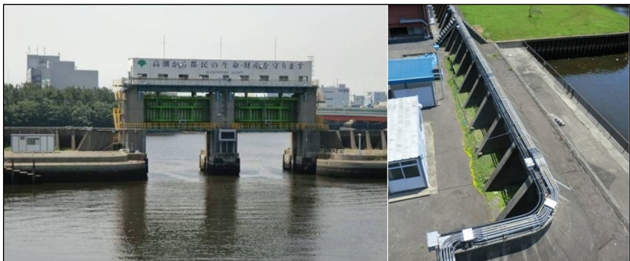
Figure 2-5: Floodgates and walls in Tokyo Bay (S.N. Jonkman, 2014)
