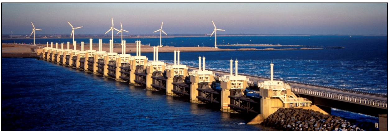
Figure 2-13: Eastern Scheldt storm surge barrier (Source: www.architecture.about.com ).
