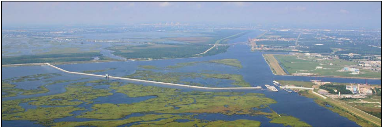
Figure 1-2: New Orleans storm surge barrier (U.S. Army Corps of Engineers, 2014).
