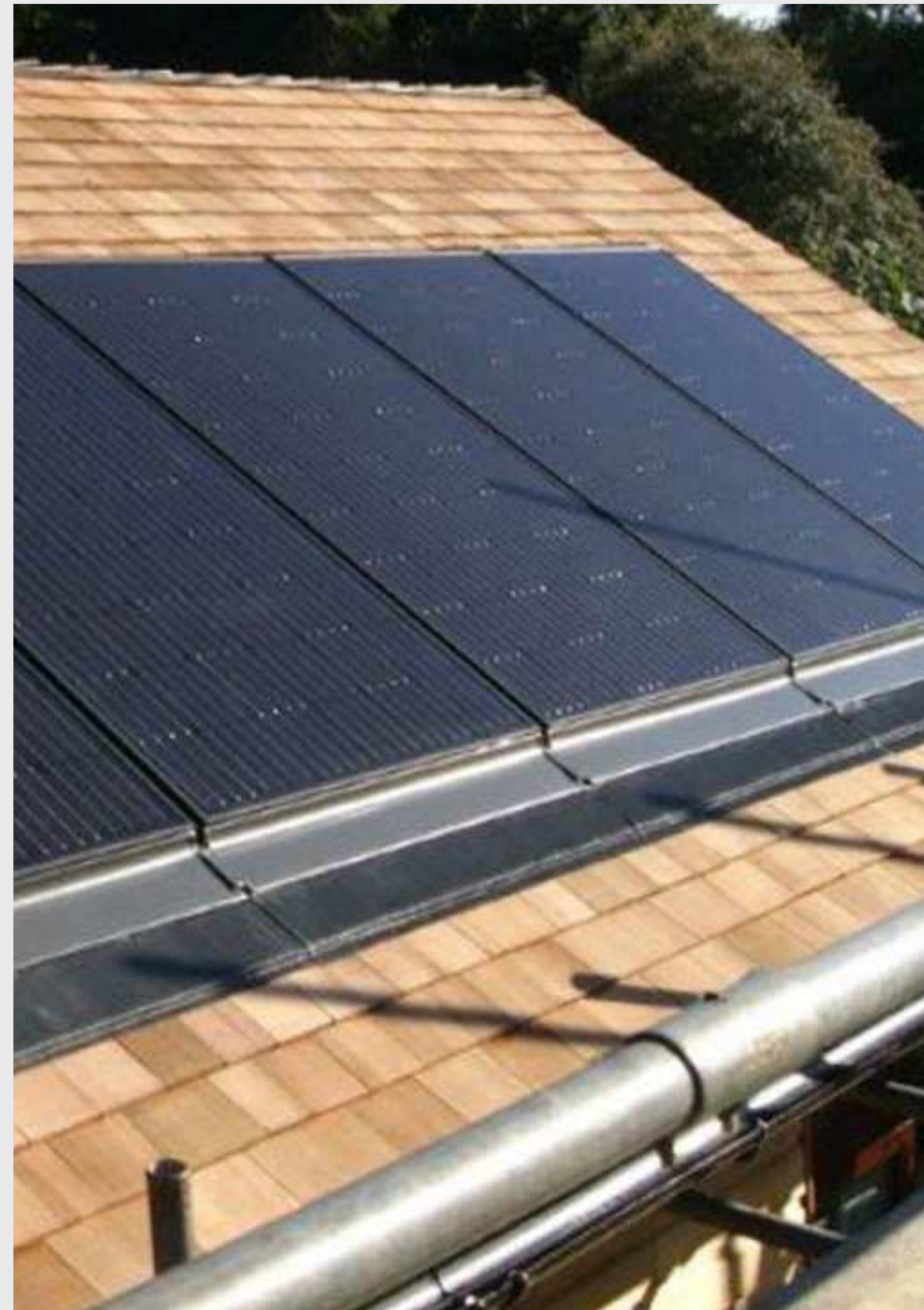
Shingle roof + PVT application Reference
