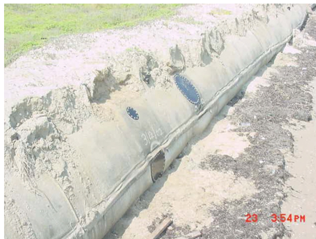
HDPE repair plates for a Geotube [HEILMAN & HAUSKE, 2003]
