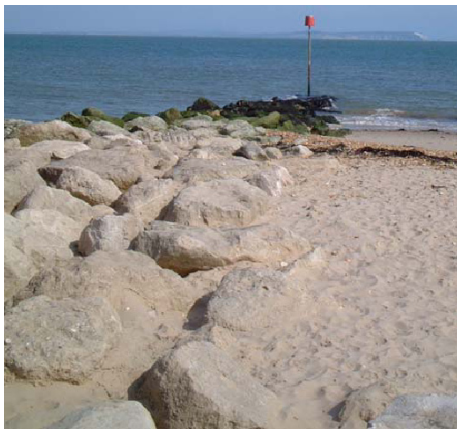
Simple groyne at the southern UK Coast, and toe detail [CROSSMAN ET AL. , 2003]
