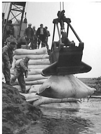
Nylon bags used for the closure of the Pluimpot, November 1957 (photo Cas Oorthuys, rvd)
