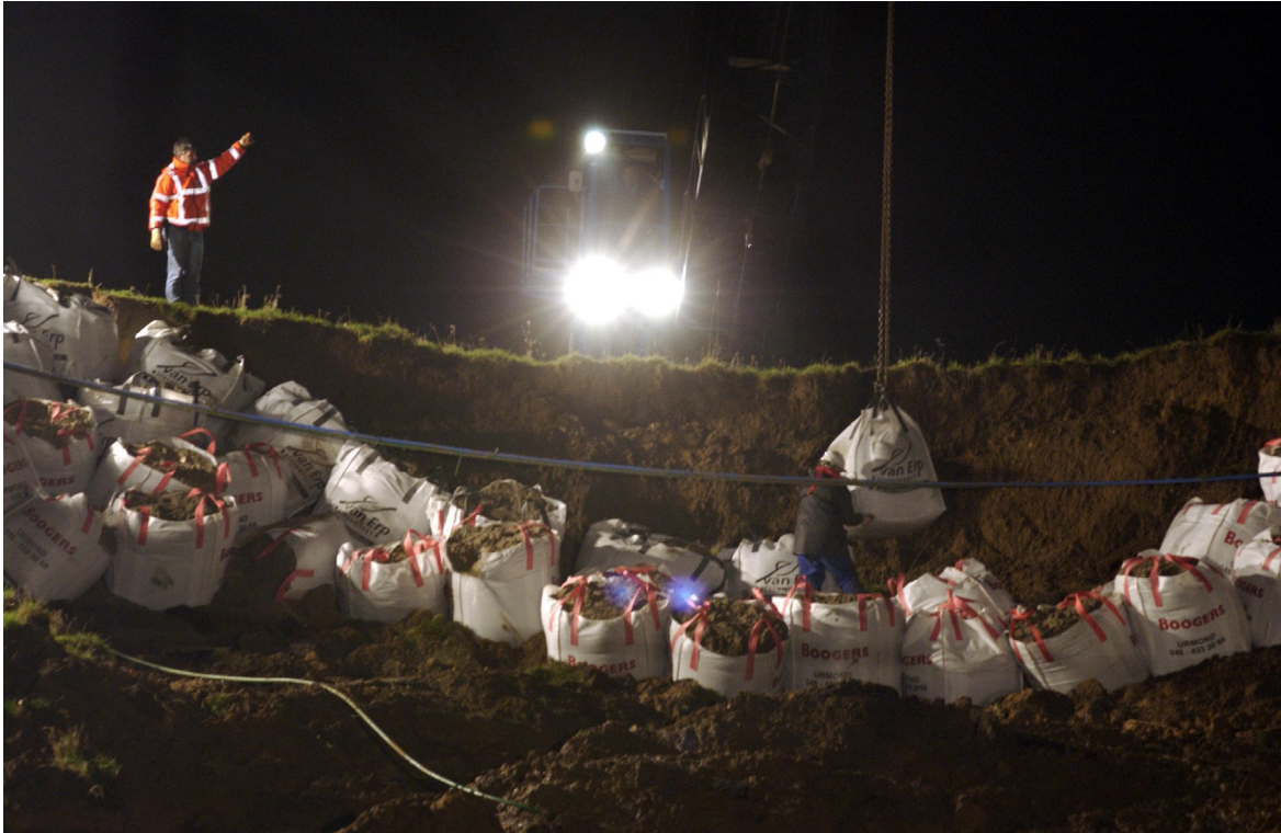
Emergency works at a dike breach in the Julianakanaal in the Netherlands, January 2004 (photo Michiel Wijnbergh/Hollandse Hoogte)
