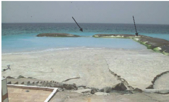
Slumping of a Geotube after a small storm in Dubai [WEERAKOON ET.AL. , 2003]
