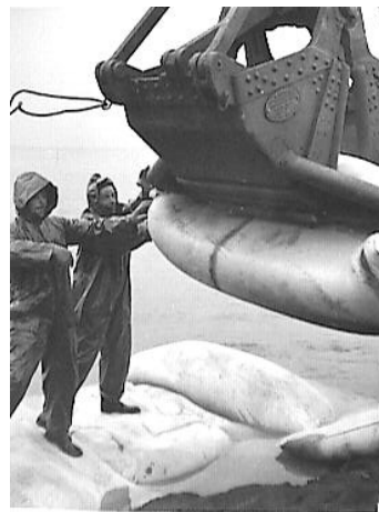
Nylon bags used for the closure of the Pluimpot, November 1957 (photo Cas Oorthuys, rvd)
