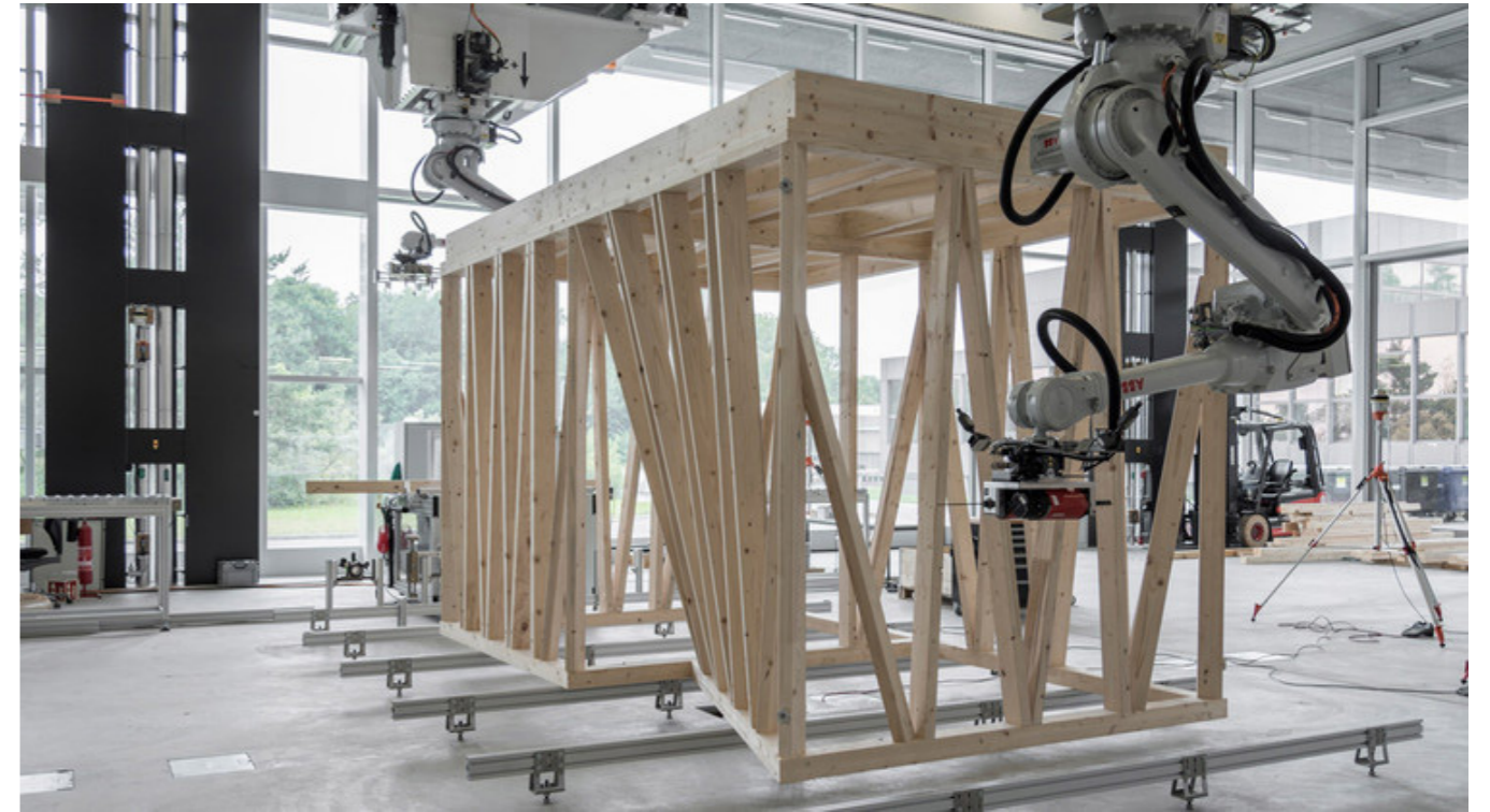
Figure 9.1 Spacial timber assembly (ETH Zurich)
