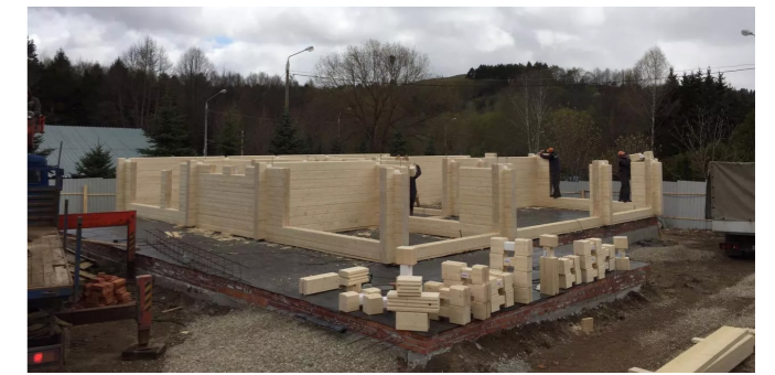
Figure Ecohousemart log construction (Ecohousemart)
