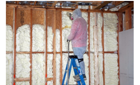
Figure Sprayed insulation (ultimate radiant barrier)
