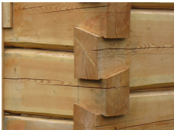
Figure Dovetail log construction (stonehouse woodworks)
