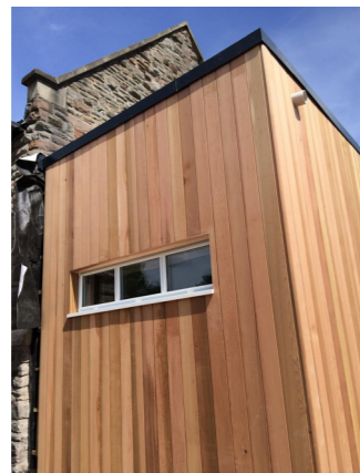
Figure Vertical closed facade cladding (Spahaus timber)
