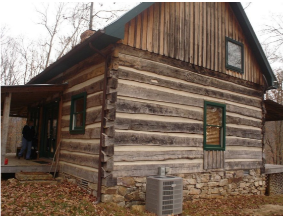
Figure Modern log construction with dovetail joint (small-cabin.com)
