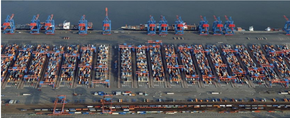
Figure 4: Overview of HHLA container terminal in Hamburg. Source: ABB (2012)
