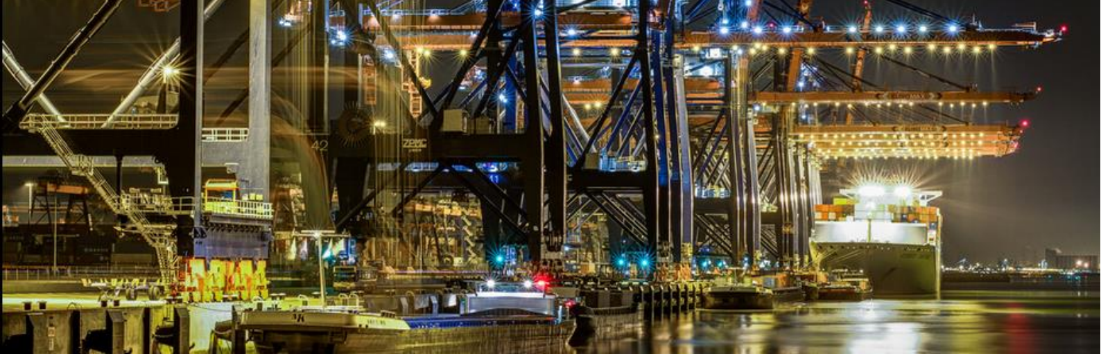
Barges and large containership docked at the Euromax terminal, Port of Rotterdam
