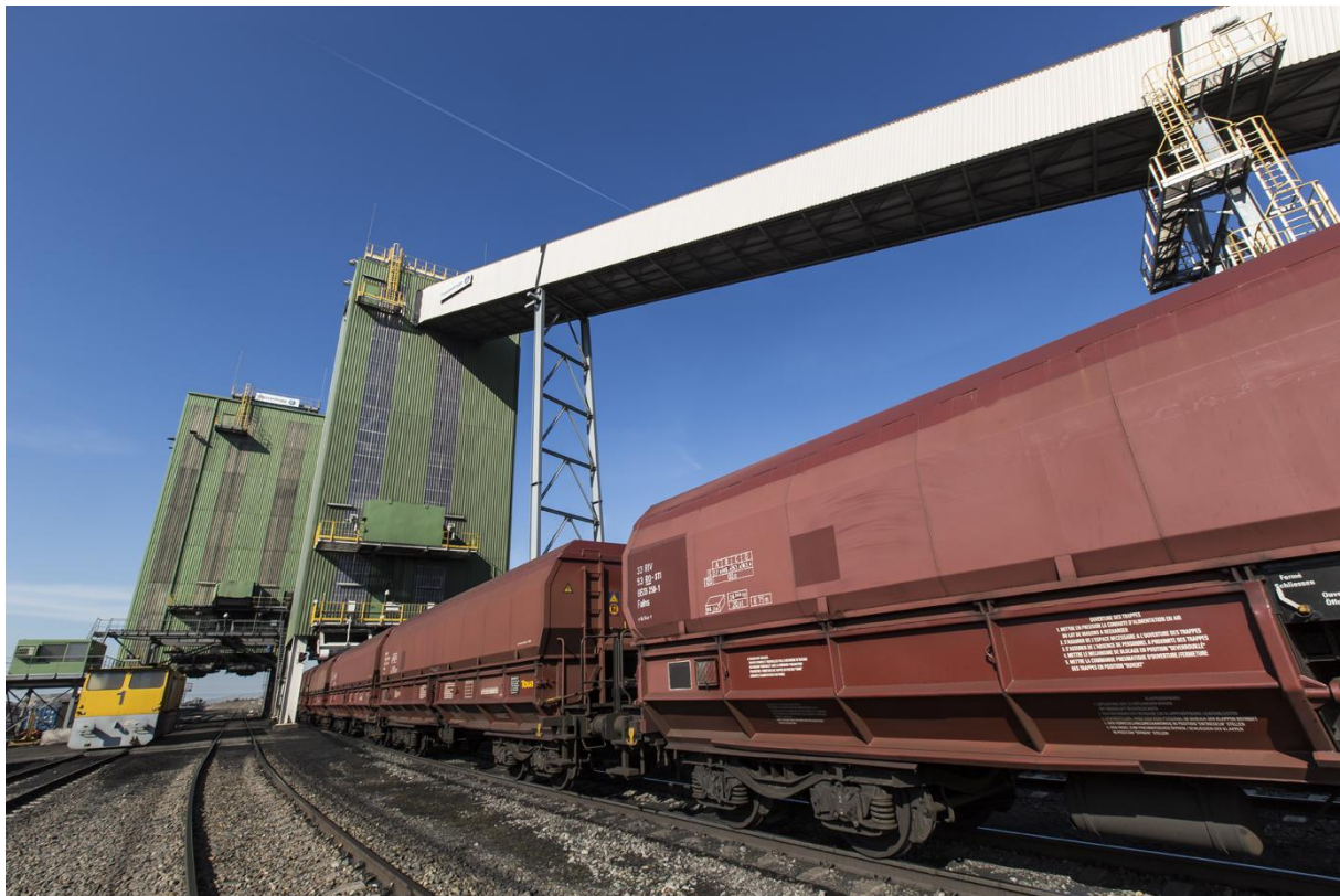
Figure 4.4: Railcar loading machines (Courtesy of EMO BV)
