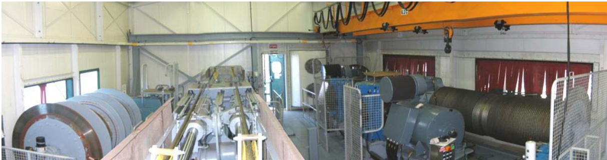
Figure 3.7: Overview of the machinery room of an STS-crane with an anti-slag device as shown in Figure 3.3. In the center the anti-slag device is visible, on the right the main hoisting winch (source: Cargotec)
