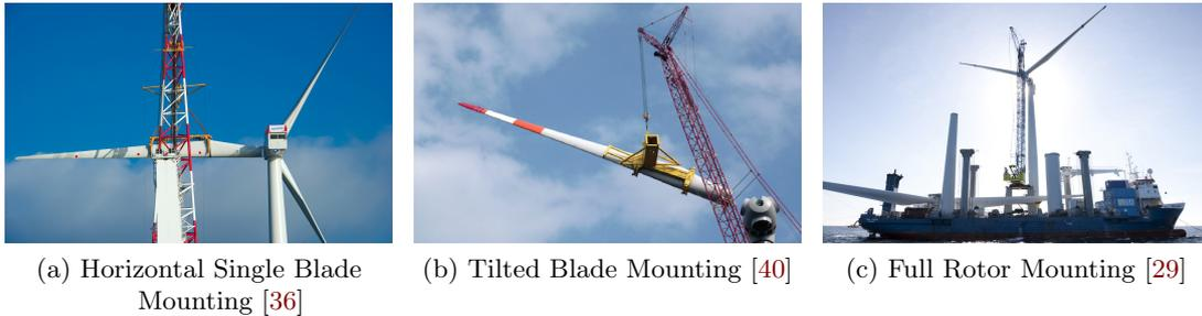
*Figure 2.1: Different Blade Mounting Techniques*
