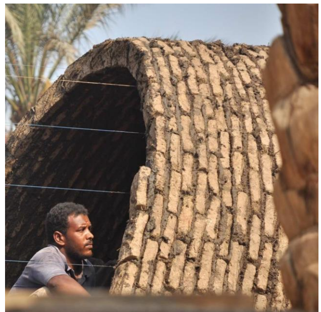
Fig. 3.20. Nubian vault construction (Aga Khan Award for Architecture, 2009)
