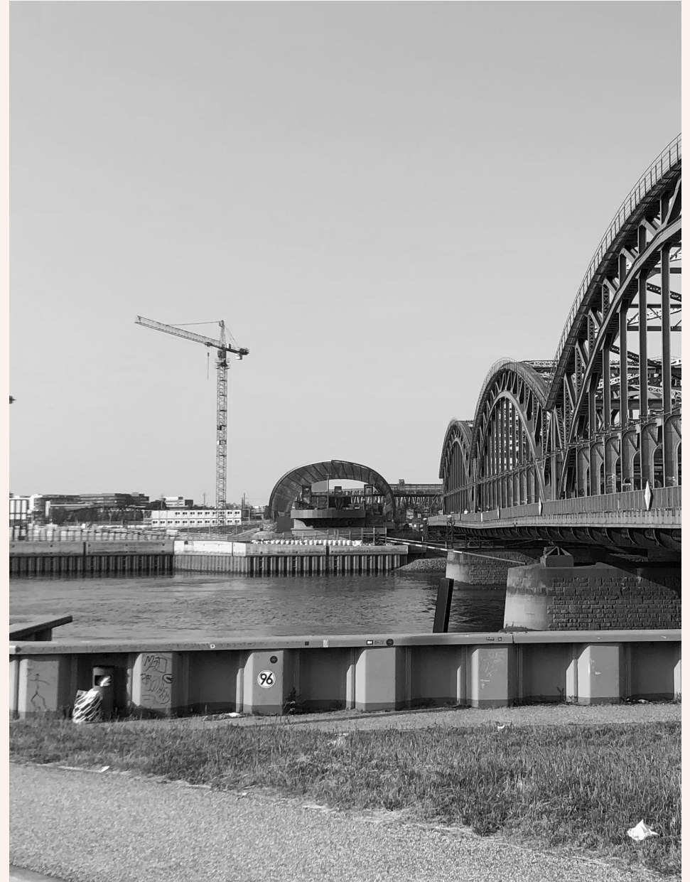
View to Train Stop Elbbrücken
