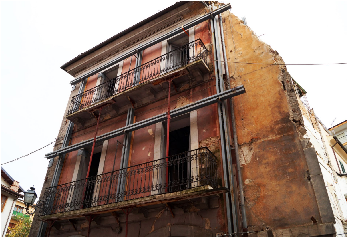
L'Aquila, shoring up, October 2016, picture by the Author
