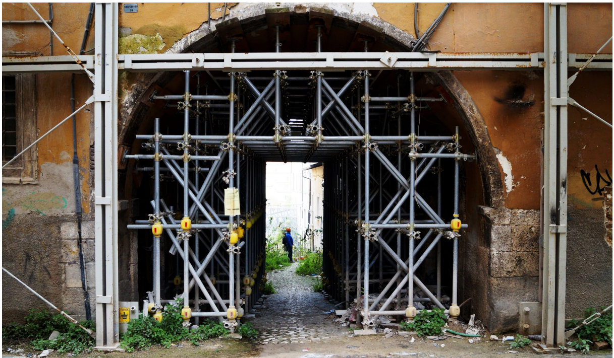
L'Aquila, shoring up, October 2016, picture by the Author
