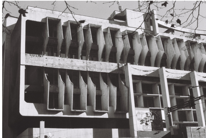
12. Soviet Modernist building in Tbilisi, Georgia
