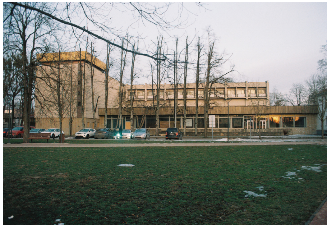
5. Abandoned building in the centre of Druskininkai. Photo by author
