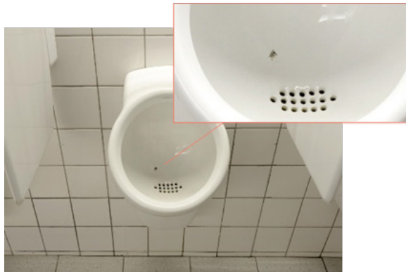
Figure 10: Urinal with a fly to aim as designed by Aad Kieboom (Evans-Pritchard, 2013).
