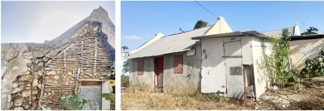
FIG. 5.1 (A) Layered housing approach observed in a historic home in Aruba. Initially constructed using wattle and daub techniques, later reinforced with concrete. (B) The same home from the opposite side, showing a newer annex constructed with wooden panels.
