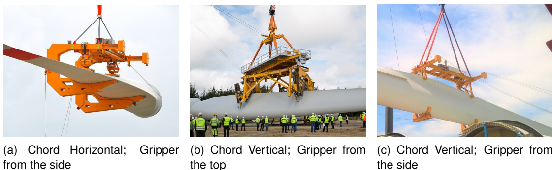
Figure 3.9: Possible combinations of Blade Buffer and Pickup Blade
