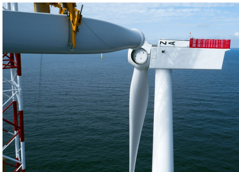
(b) Lineup of a blade with a hub [30]
