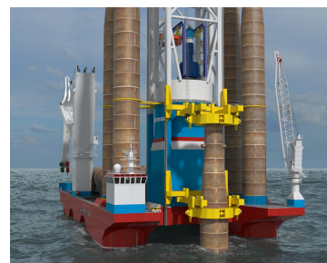
(c) Lower Monopile to Seabed
