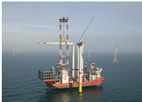
(a) Lift blade to hub height
