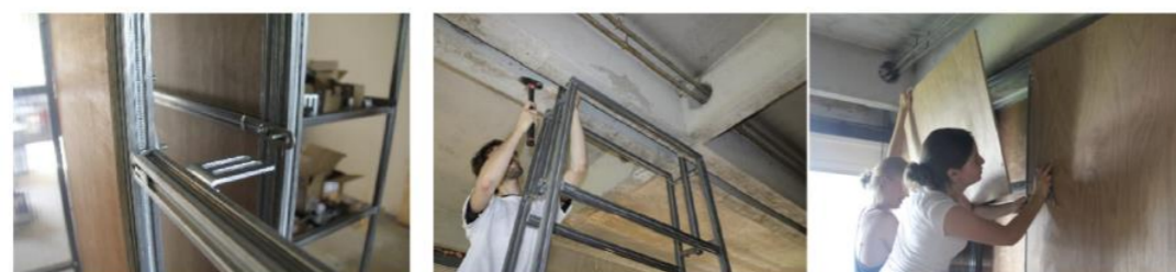
Figure 5. The steel frame wall with plywood panels.
