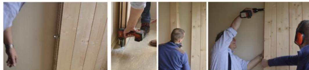
Figure 4. The massive wood interior partition wall.
