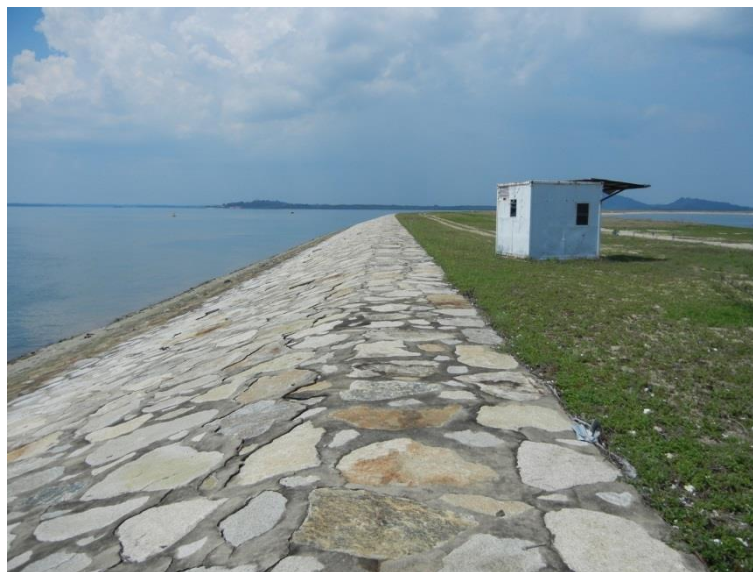
Figure 4.14: Cemented armouring of the armour layer on the existing sea dike of Pulau Tekong.
