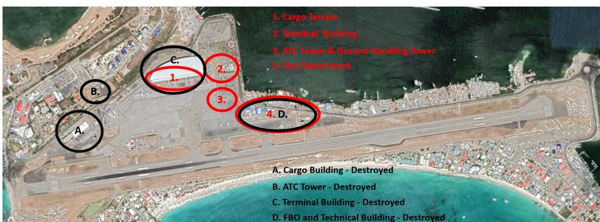
Figure 2.5: Princess Juliana International Airport General Lay Out after Irma [23].
